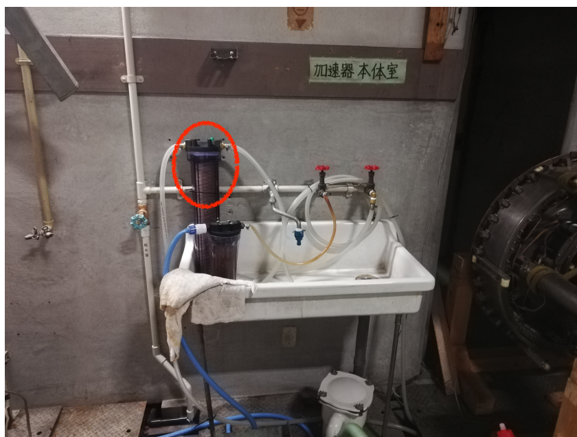
Figure 4.8: Water filter and water supply for cooling TMP pump and compressor.
